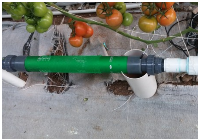
Installation at a Mexican tomato grower.
