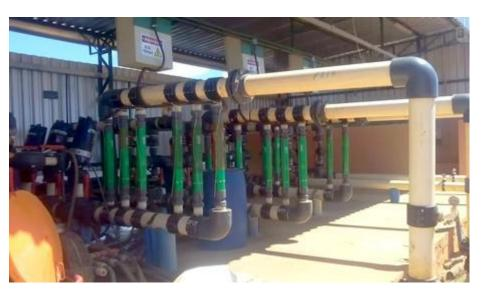
The system uses a finely calibrated electromagnetic signal to treat irrigation water before it is applied to crops. The system dissolves minerals and other organic material in the water into smaller elements, immediately improving any plant's ability to better absorb what it needs in the proper proportions.
